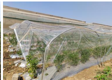
Construction of barrier
